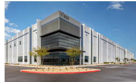
LITCHFIELD LOGISTICS - BUILDING 3 SURPRISE, AZ SIZE: 324,800 SF
